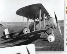
The 1918 Sopwith Snipe was the successor to the Camel with a more powerful Bentley rotary engine. It was the RAF's front line fighter until 1926
