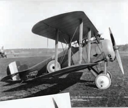
**The 1918 Sopwith Snipe was the successor to the Camel with a more powerful Bentley rotary engine. It was the RAF's front line fighter until 1926**
