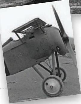
**The 1918 Sopwith Salamander TF 2 was an armoured ground attack fighter developed from the Snipe**
